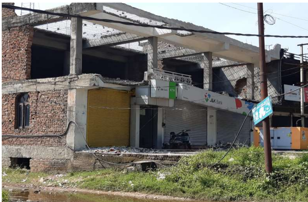
Fig. 3 Demolishing of Buildings on the Jammu-Akhnoor Highway
