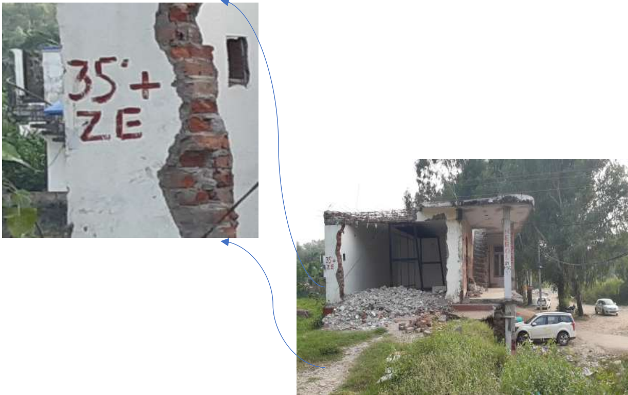
Fig. 7 Markings by Govt. Officials to demolish the construction
